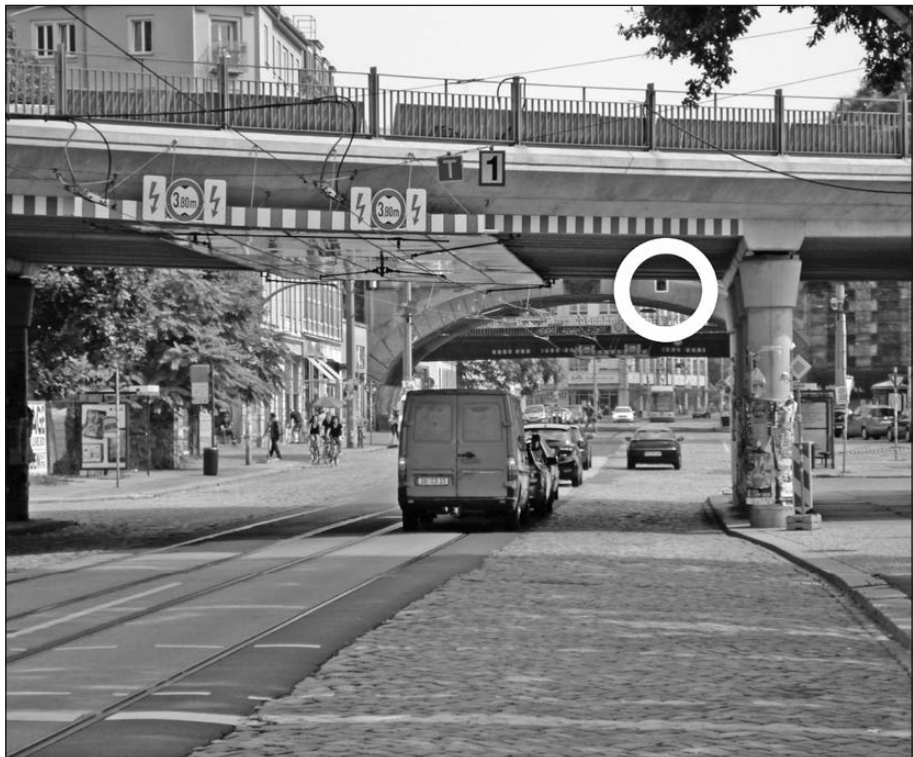
Figure 68: Traffic light concealed by bridge (lower half marked with yellow circle): Advance warning signs must be used in this situation (picture shows a situation in Dresden) (picture: Weller).
