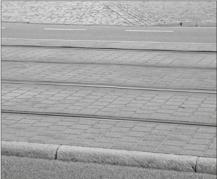
Figure 69: Fifty shades of grey with low contrast make it difficult for older drivers to perceive their path. Curbs and tram paths should be coloured or equipped with retroreflective materials (picture shows a situation in Dresden) (picture: Weller).
