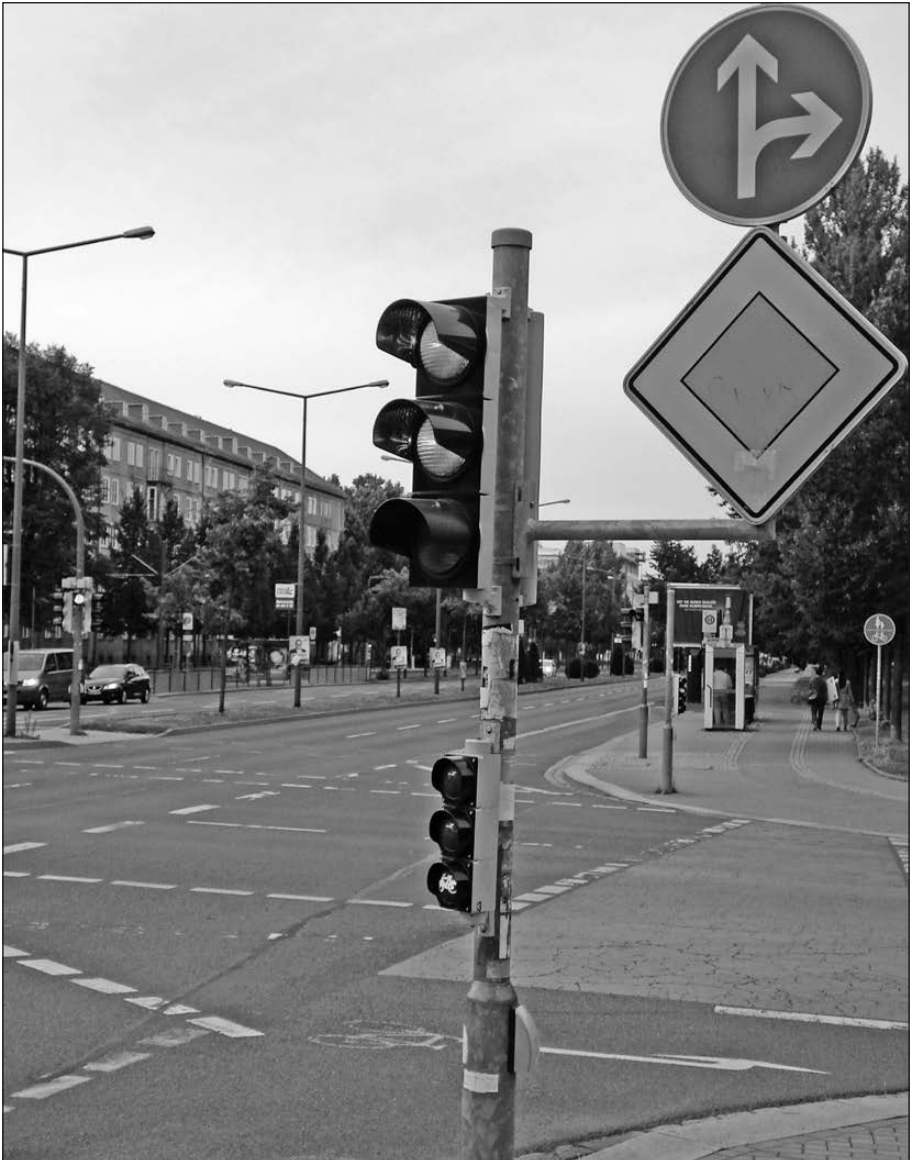
Figure 63: Traffic light with head-start for cyclists. Although this can cause ambiguity for drivers not familiar with this regulation it will probably not be dangerous as other traffic participants have a red light (example of situation in Dresden) (picture: Weller).
