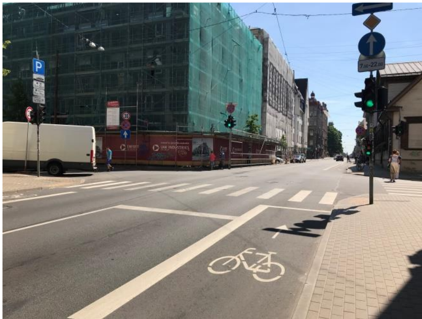
Figure 28. Cycle lane with advanced stop line at a signalised intersection, Riga
